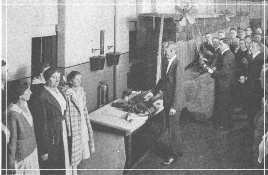
A. W. DICKINSON PULLING THE SWITCH WHICH PUT KILDARE CENTRAL OFFICE IN SERVICE
